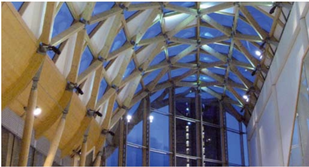
Internal view of the roof glass with the load bearing diagrid structure.
